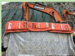
設置可移動的臨時隔音屏障 Installation of Removable Temporary Noise Barriers
